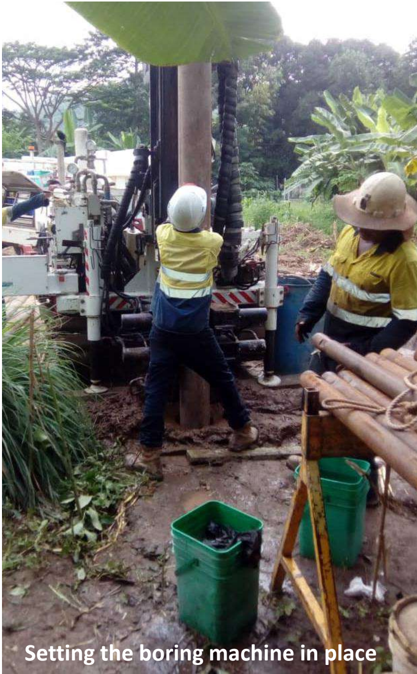
Water brought from Dili to lubricate the drill preventing it from overheating
