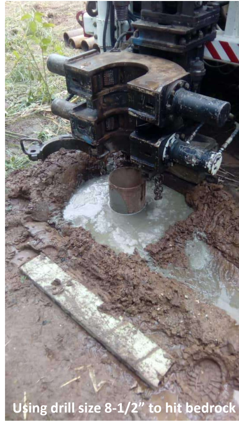
Water brought from Dili to lubricate the drill preventing it from overheating
